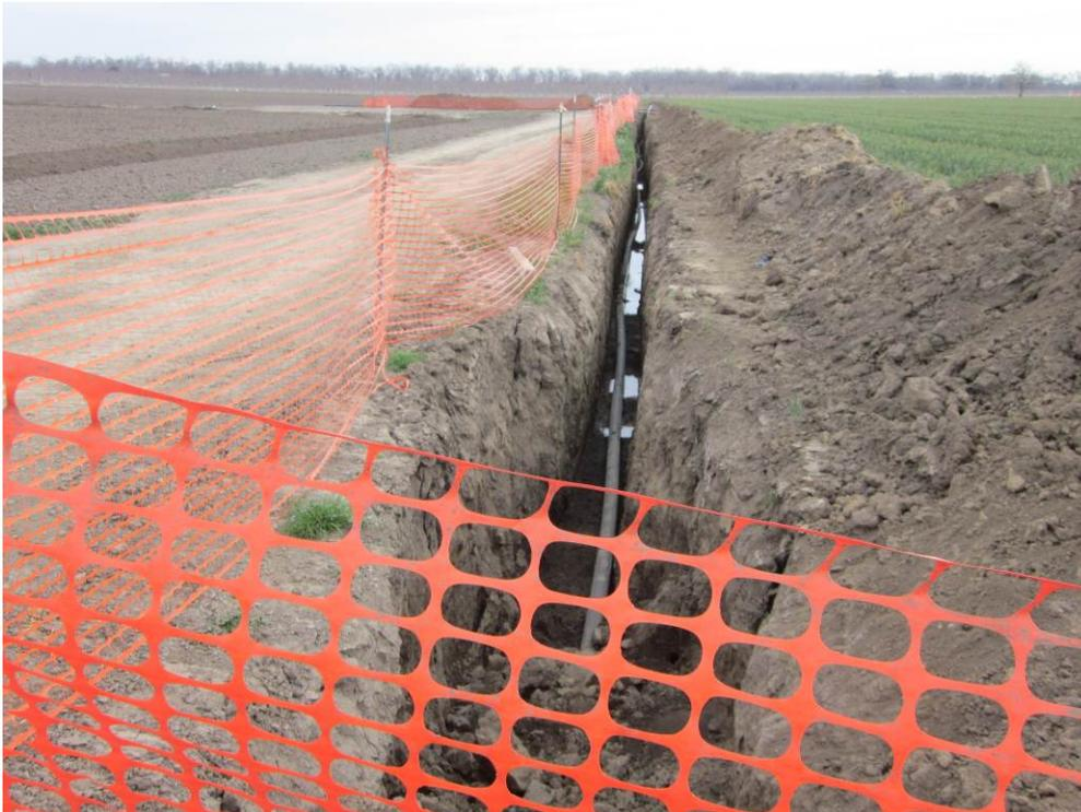
**Photo 2:** Trench for the 8-inch pipeline connecting the saltwater storage tank (at the Remote Well Pad site) and the saltwater disposal well has been completed.
