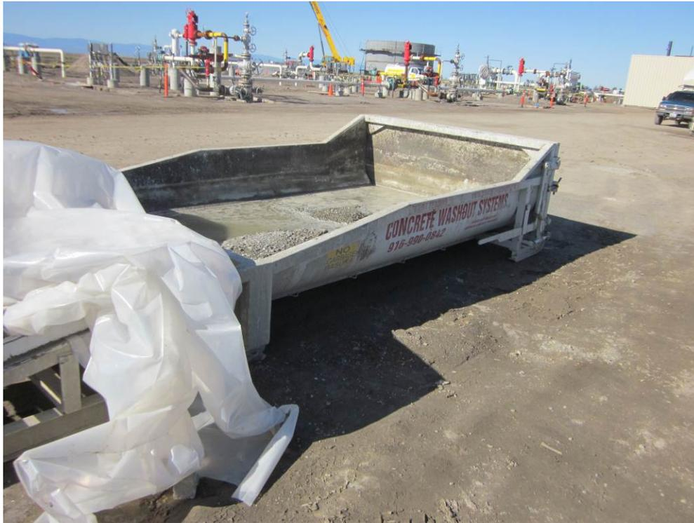
**Photo 3:** Concrete washout provided at the Compressor Station site for containment of excess concrete.
