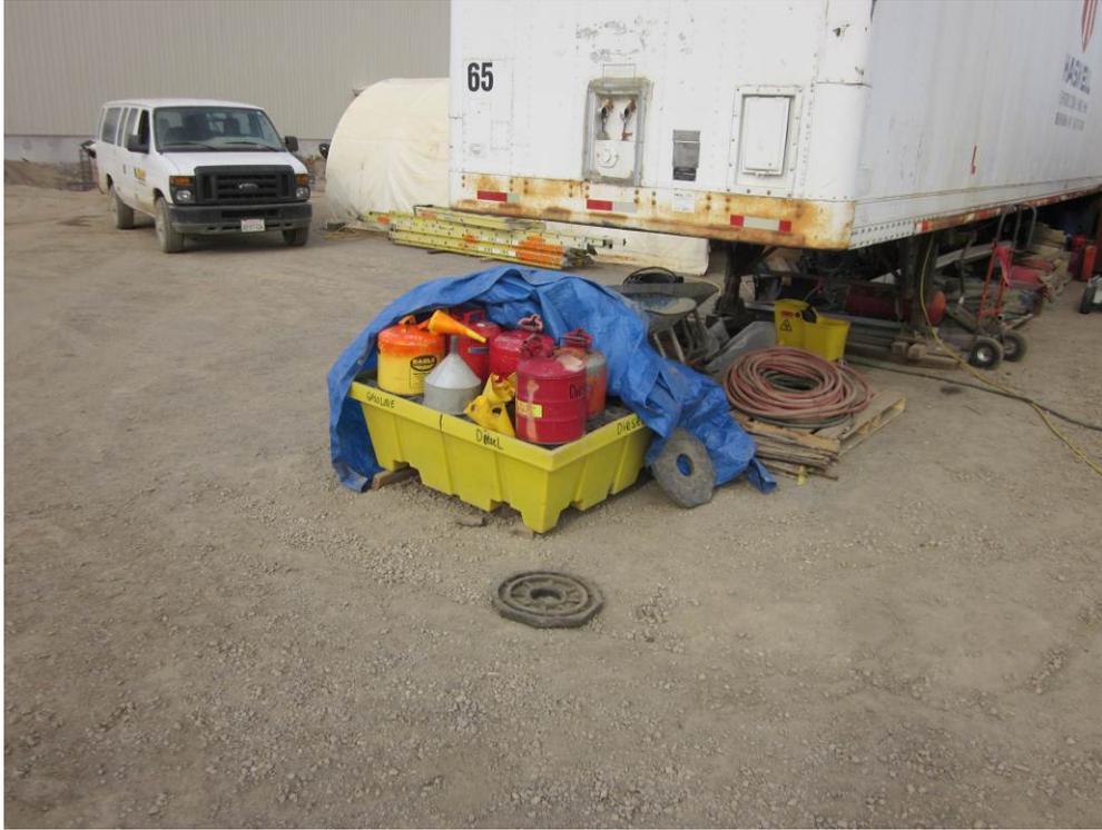
**Photo 5:** Secondary containment provided for fuel tanks at the Compressor Station site.
