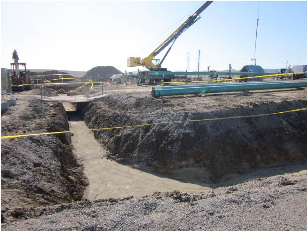
**Photo 6:** Trenching is underway at the Metering Station site for natural gas pipeline connection.
